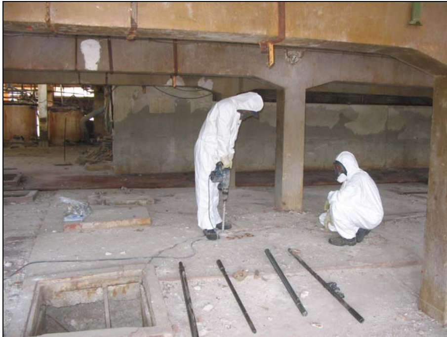
Figure 6: Sampling of construction materials in the former electrolysis plant
